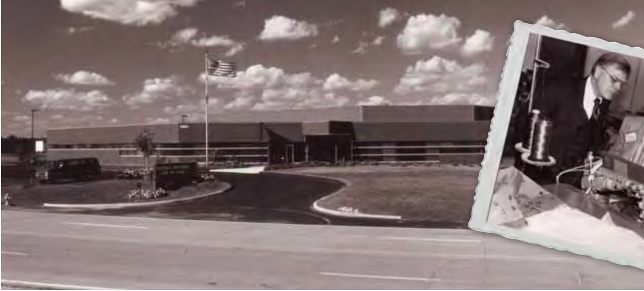
NIB's 25,000-square-foot Technical Center built in St. Louis in 1985.
